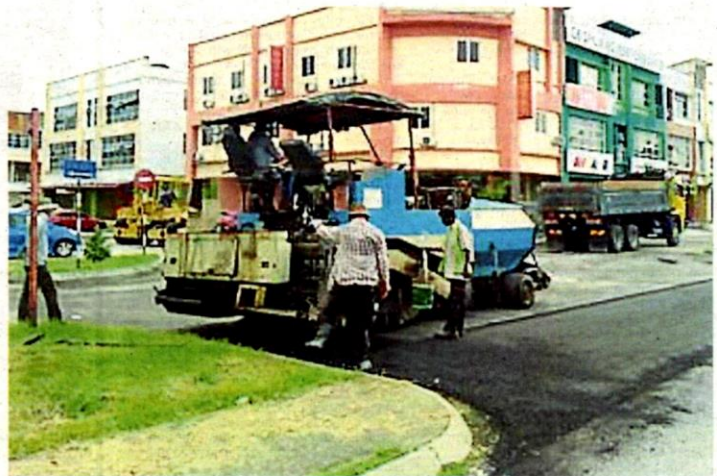
Road resurfacing work taking place around Klang Sentral bus terminal.
